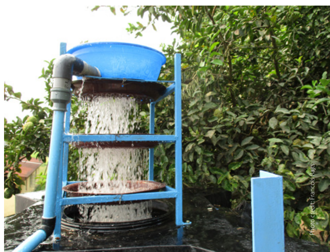
Plate 4. An aeration tower on the top of a hatchery reservoir.
