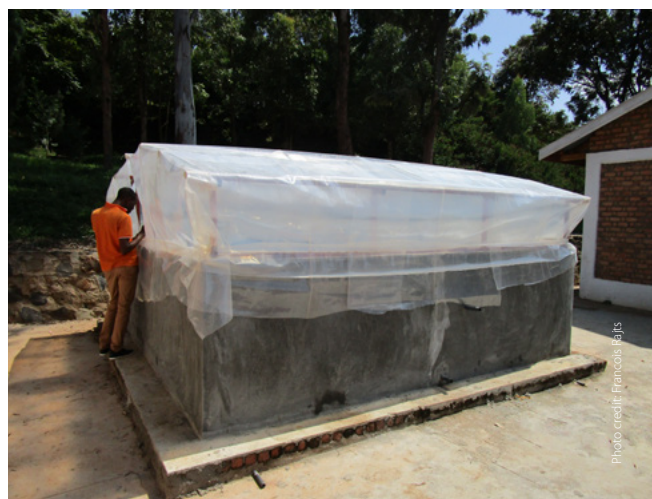
Plate 1a. A greenhouse cover on the reservoir tank provides heated water for the hatchery in Kalambo, DRC.
