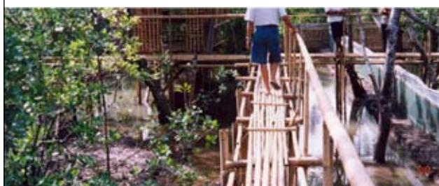
FIGURE 8.6 Mangrove pen with wooden walkway
